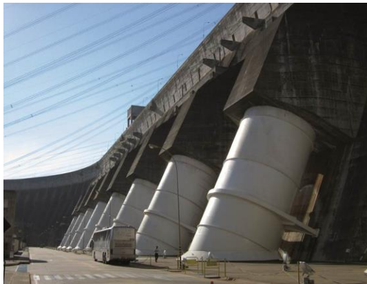
Itaipu - The biggest hydroelectric plant of the world
